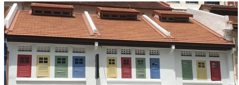
Before (top) and after (bottom) cleaning and localised one-for-one replacement of cracked tiles
