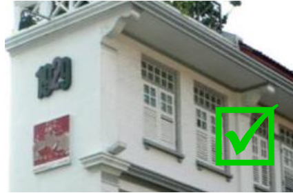
On gable end wall
