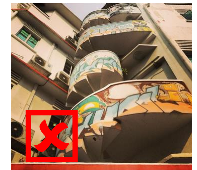
On spiral staircase – Not Allowed
