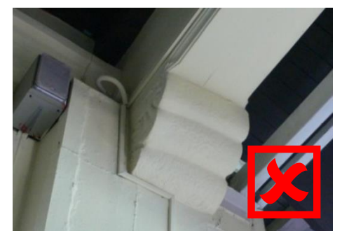
Original granite corbel
