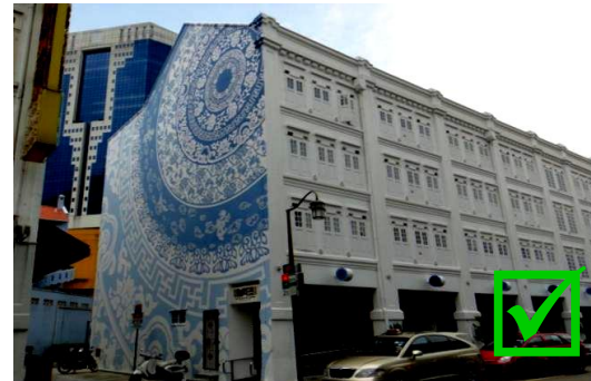
On end gable wall
